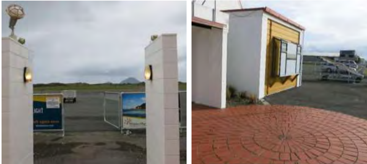
Concrete block pillars at entry(left) view west, showing entry patio
