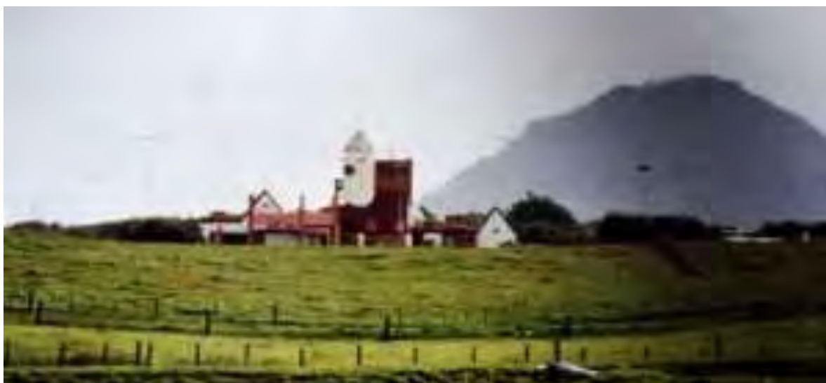
The Whakatāne airport building, with Moutohora /Whale island visible behind. Photograph: Roger Walker
