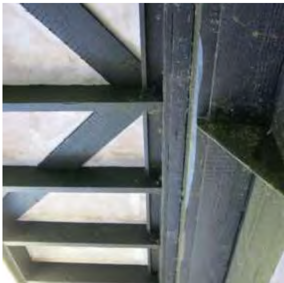
Ceiling over former open canopy (left) ceiling detail + section of wire mesh fixed to rafters
