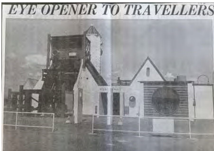
The terminal under construction. Source: Auckland University Shepard File
