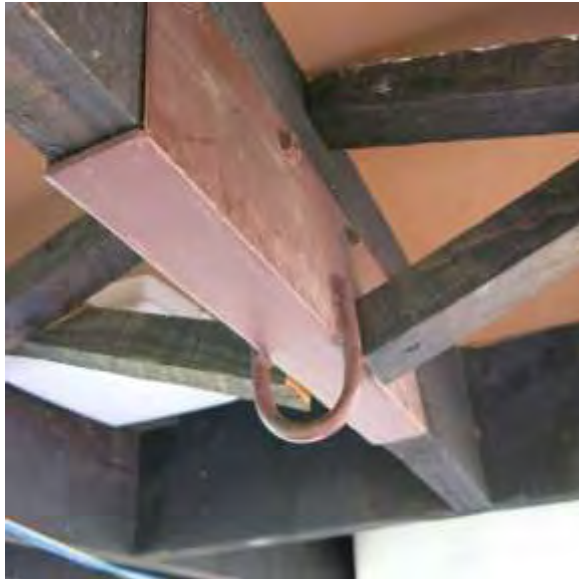
Steel winch bracket fixed to rafter (left) exposed ceiling structure +bulkhead light fittings, 1 x original
