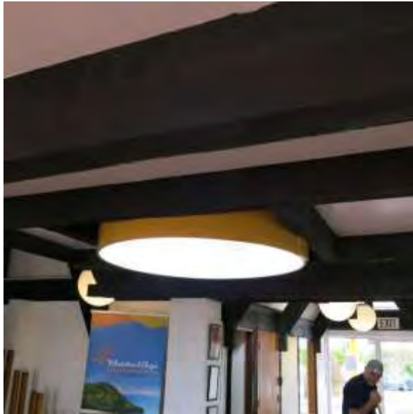
Sewer pipe skylight in flat section of ceiling (left) pipe window in north wall
