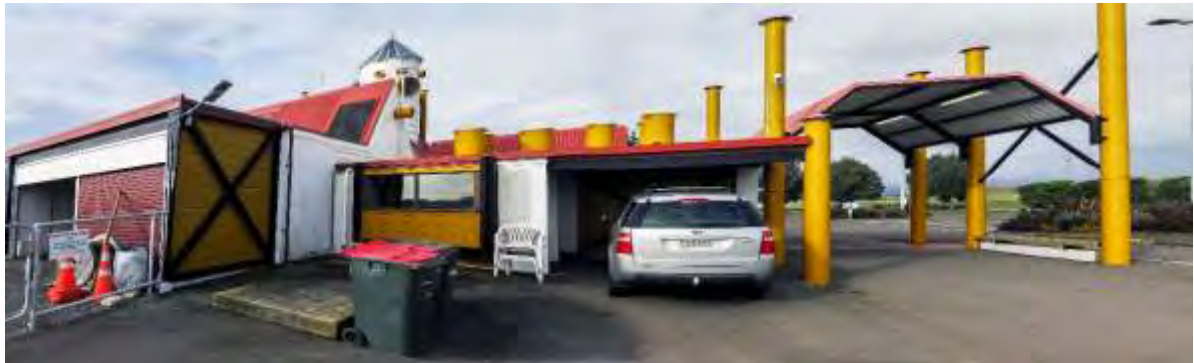
West elevation. Photograph: Graeme Burgess 2016
