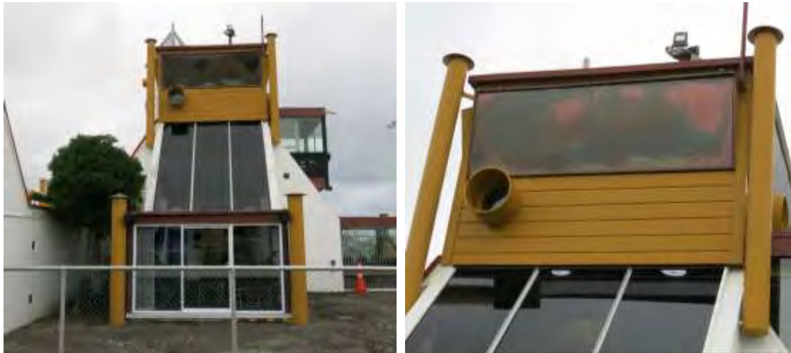
East elevation, control tower details. Photograph: Graeme Burgess 2016
