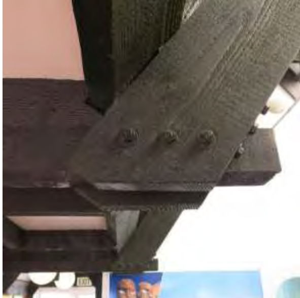
Beam + rafter detail (left) view looking up to ceiling
