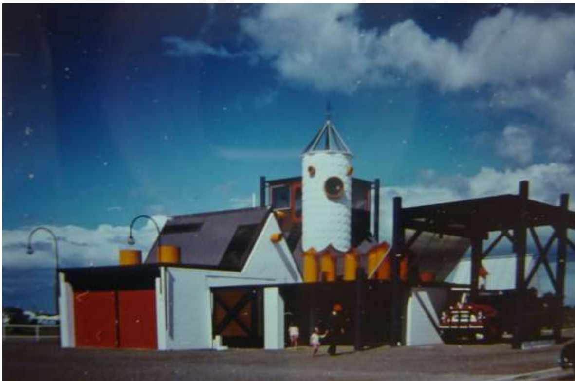
Photograph of terminal taken shortly after opening. c. 1974 Source Archives NZ Reference No. AEPK W2774 20231 Box 7
