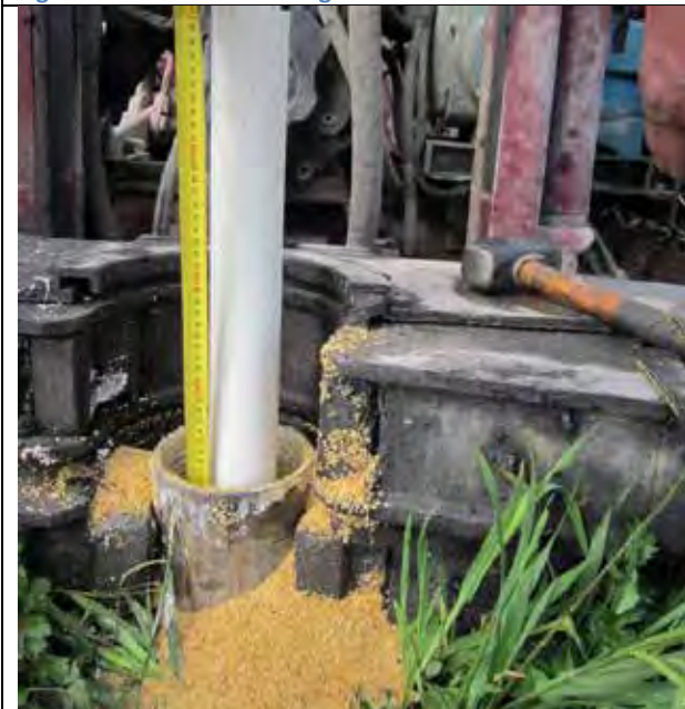
Figure 31 silica sand gravel pack
