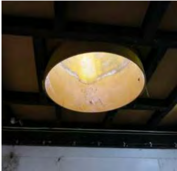
Sewer pipe skylight (left) showing ceiling in baggage room, unpainted hardboard panels
