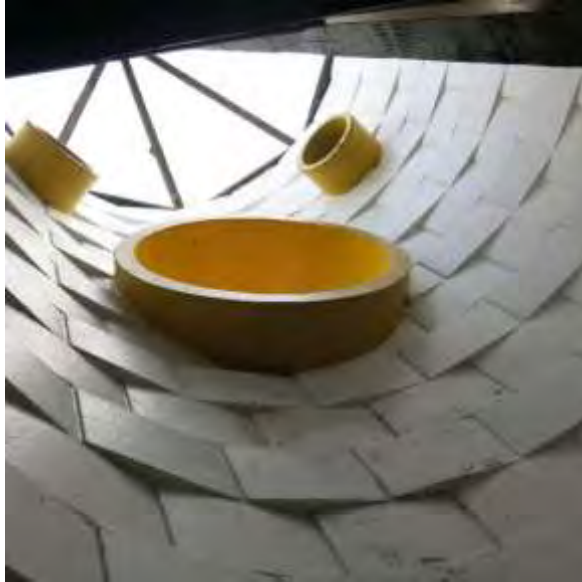
Pipe windows in stair turret (left) view up to glazed conical roof in turret
