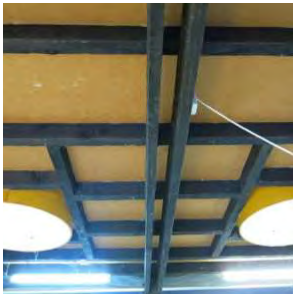
Showing ceiling with 2 x sewer pipe skylights (left) wire mesh fixed to rafters
