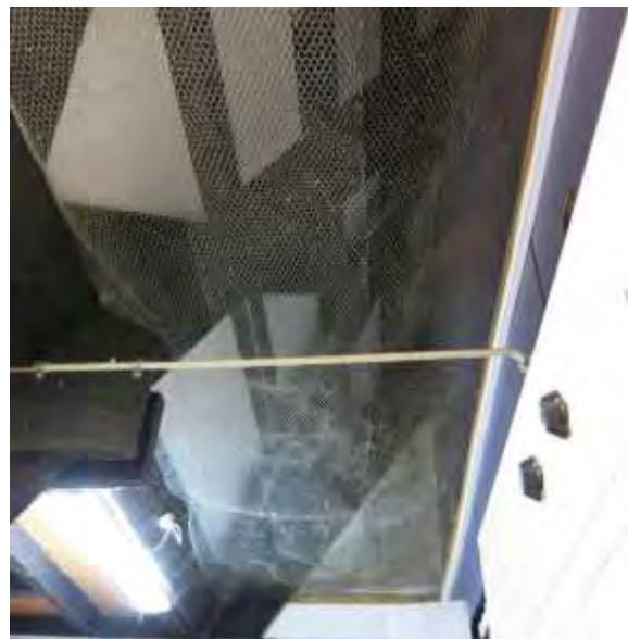
Ceiling over former open canopy (left) ceiling detail + section of wire mesh fixed to rafters
