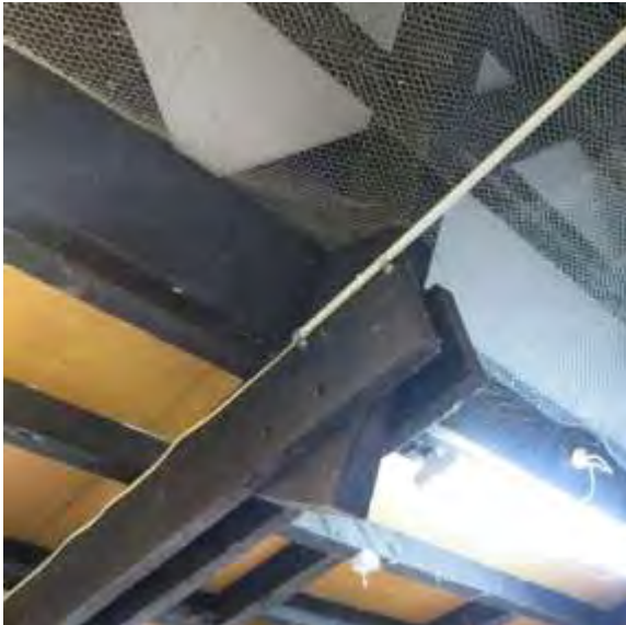
Ceiling over former open canopy (left) ceiling detail + section of wire mesh fixed to rafters
