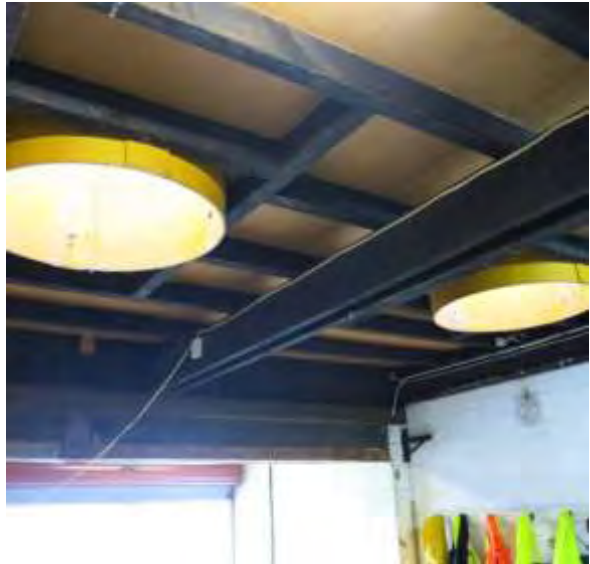
Sewer pipe skylight (left) showing ceiling in baggage room, unpainted hardboard panels
