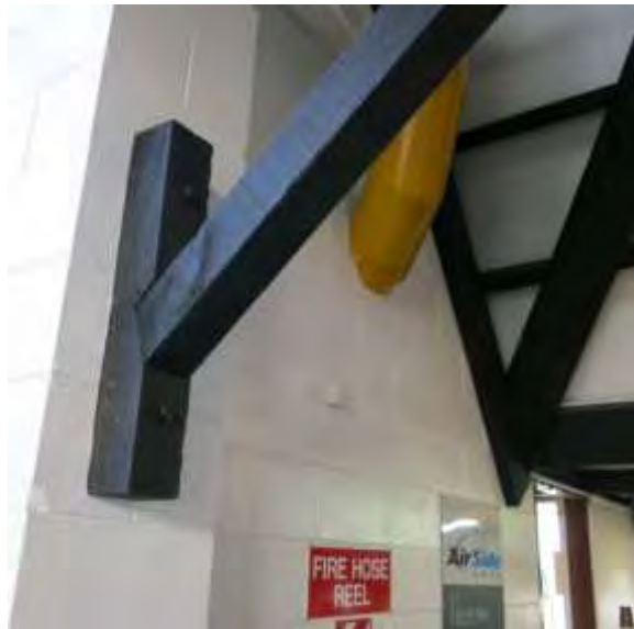
Showing ceiling + east wall with services duct penetrating (left) bracket + pilaster detail, east wall
