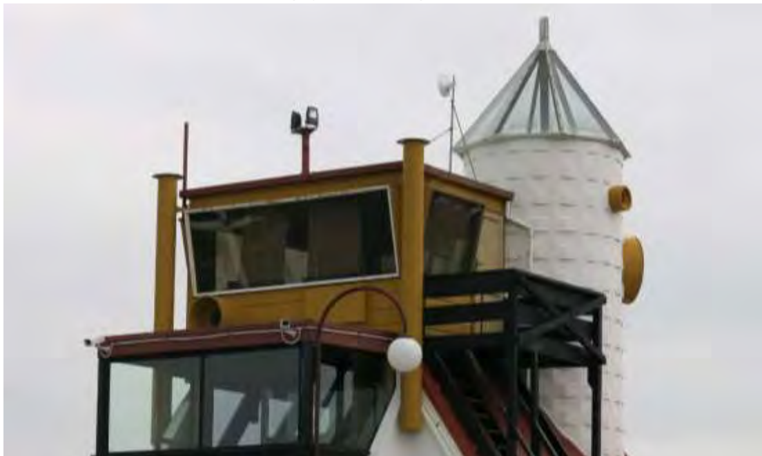
Control tower, north west corner. Photograph: Graeme Burgess 2016
