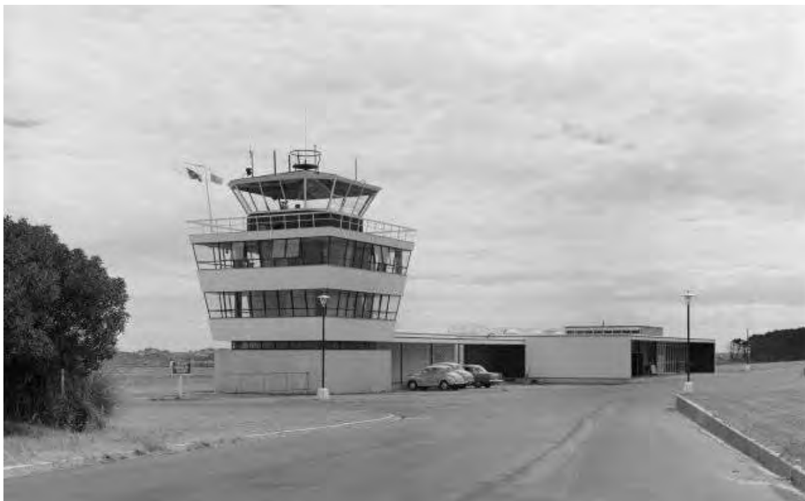
Control tower at Wanganui Airport. Photograph taken by Duncan Winder between circa 1962 and 1970. Image: Alexander Turnbull Library, Reference Number: DW-0487-F
