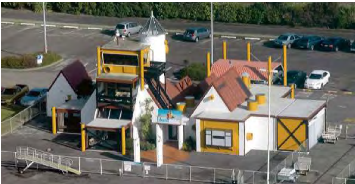
The terminal building. Source: http://Whakatānebeacon.co.nz/2014/11/air-nz-withdrawal-threatens-jobs/
