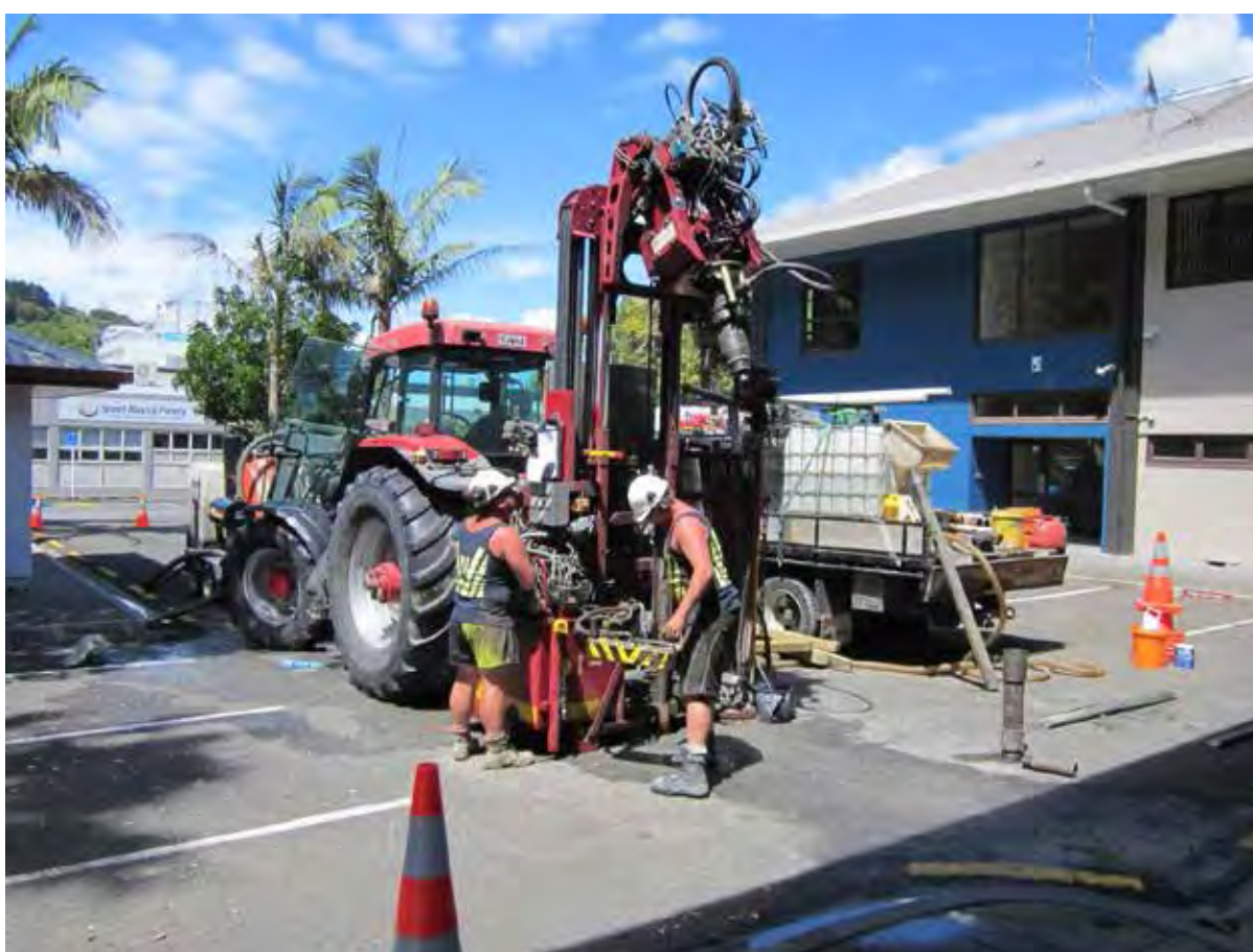
Figure 1. GEOTECH sonic rig, BH 17 Mayors carpark
