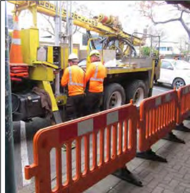
Figure 19. GEOTECH CPT rig on Strand, note pedestrian management
