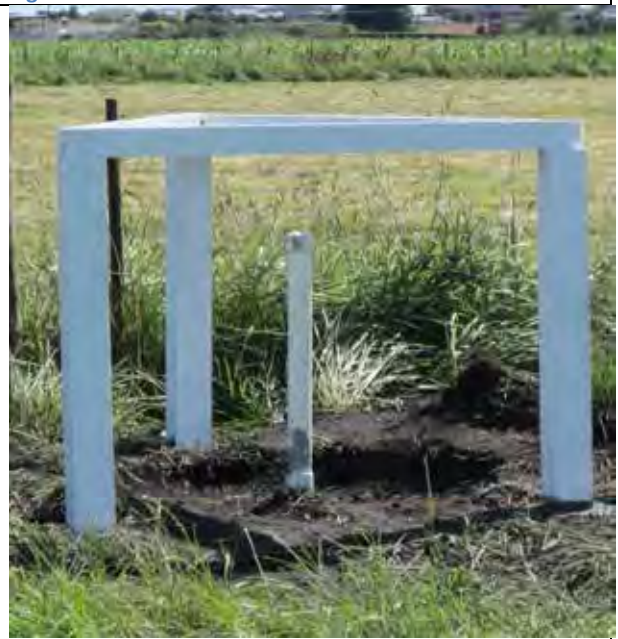
Figure 32 upstand prior to enclosing in monument
