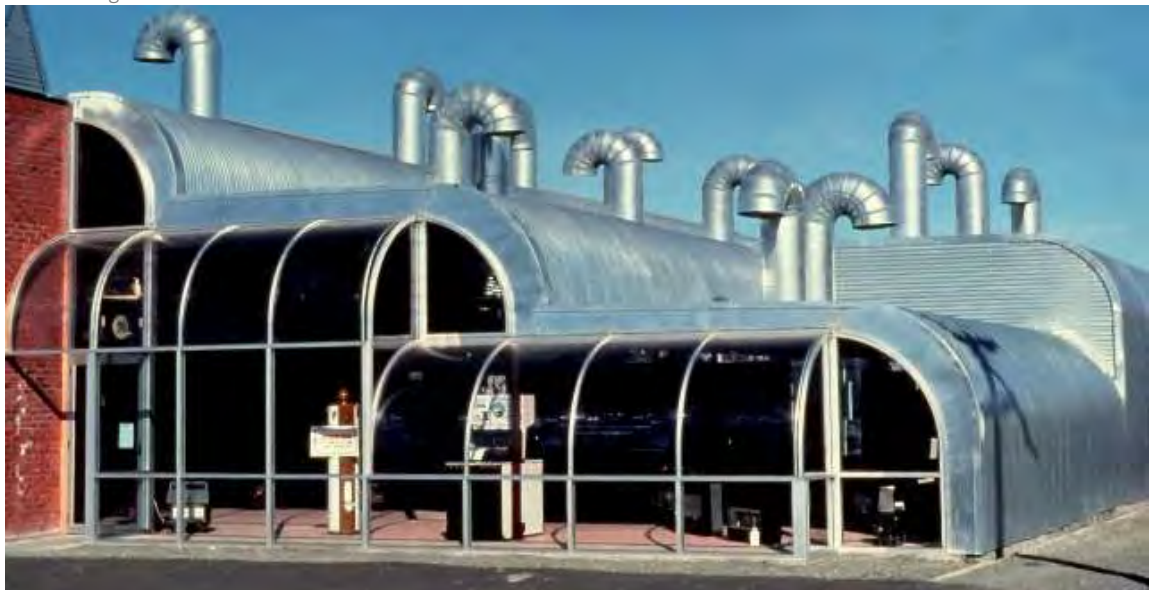
Gas House Gisborne. Gas appliance retail and service store. Corrugated roofs used as bracing. Source: Roger Walker
