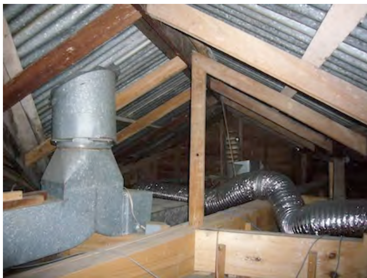
Roof Space (August 2009)
