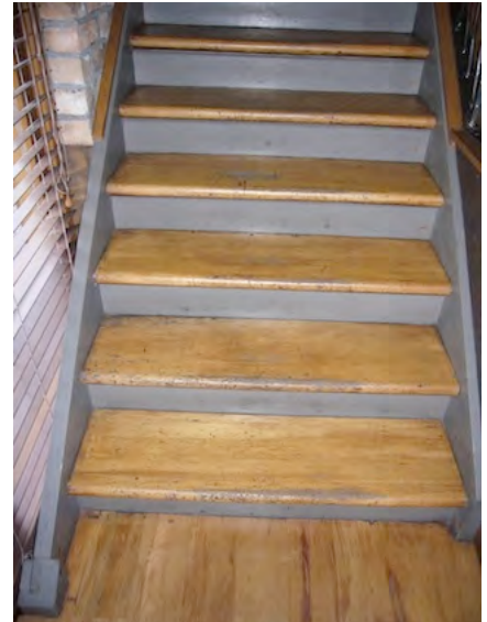
Detail of relocated Stair (August 2009)
