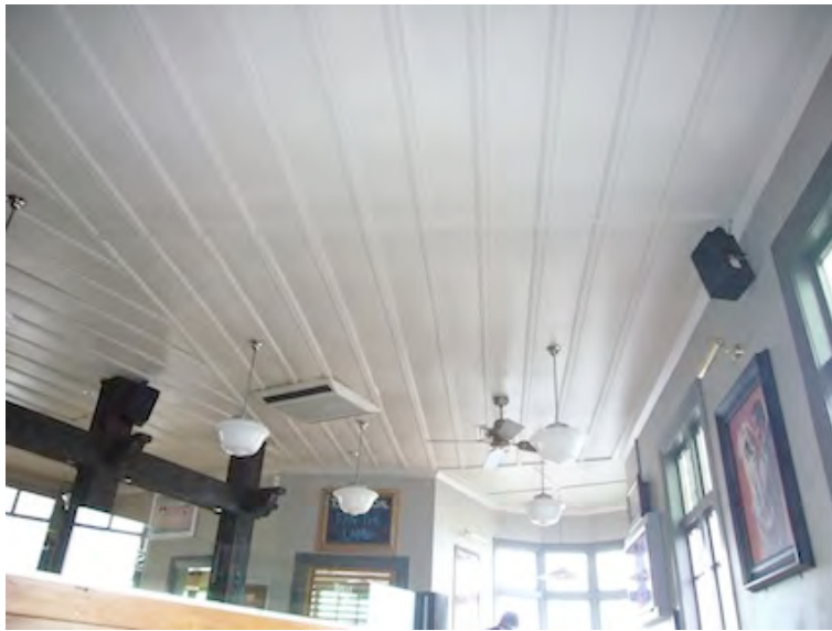
Upper Floor Ceiling (August 2009)
